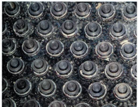
Studs are installed in a matrix pattern
